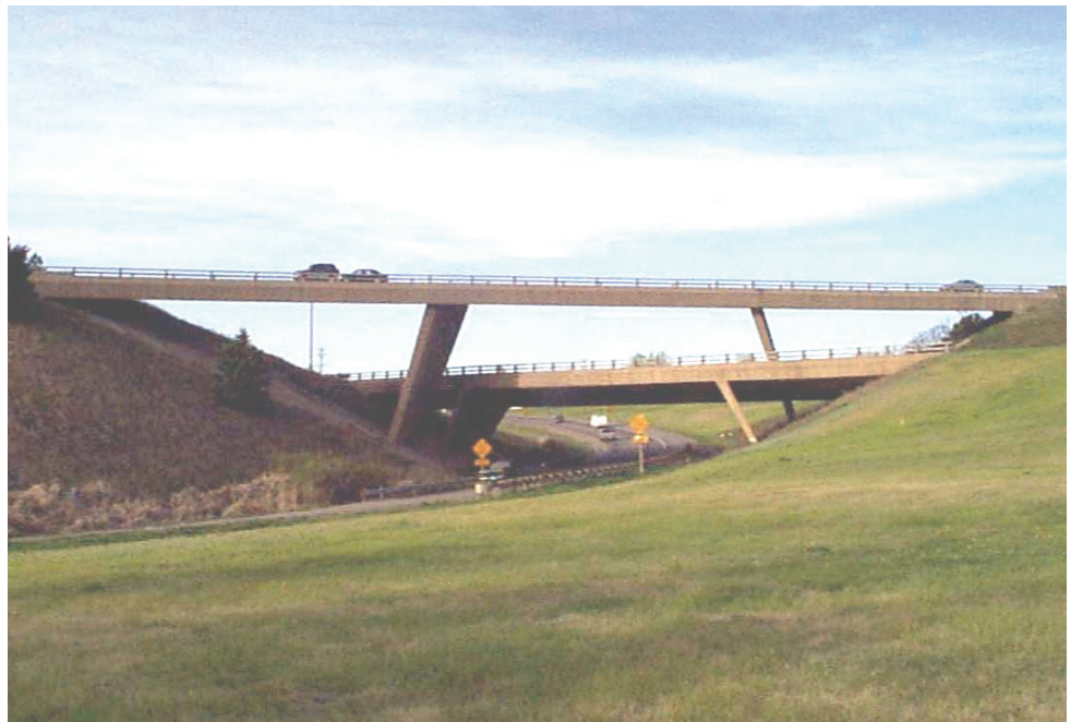
Figure 7.6.1 Three Span Concrete Rigid Frame Bridge
