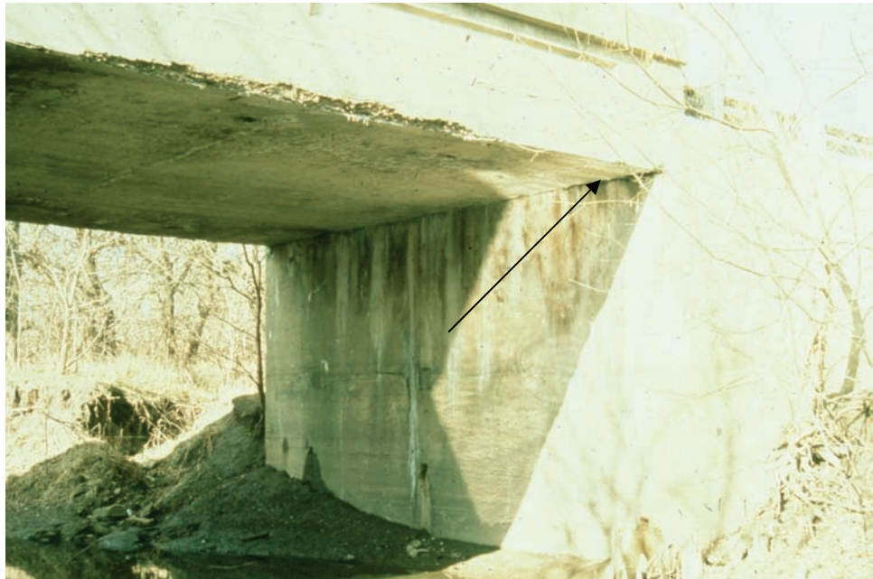
Figure 7.3.6 Bearing Area of a Through Girder Bridge
