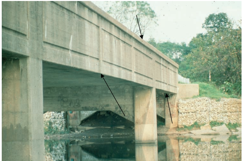
Figure 7.3.7 Typical Elevation View of a Through Girder Bridge with Tension Zones Indicated
