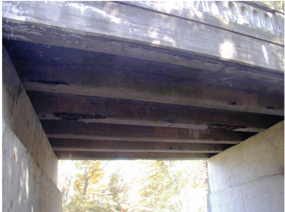
Figure 7.2.1 Simple Span Tee Beam Bridge
