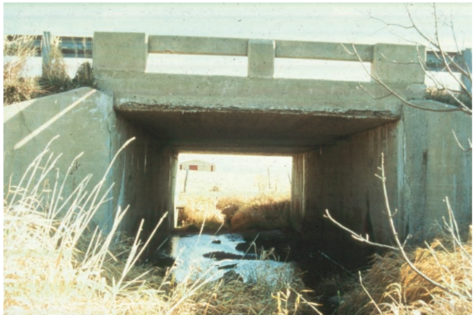
Figure 7.1.1 Typical Simple Span Cast-in-Place Slab Bridge
