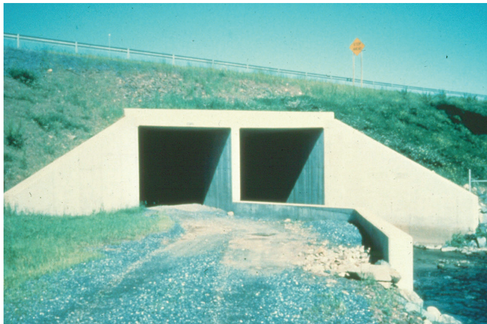
Figure 7.6.3 Typical Concrete Frame Culvert
