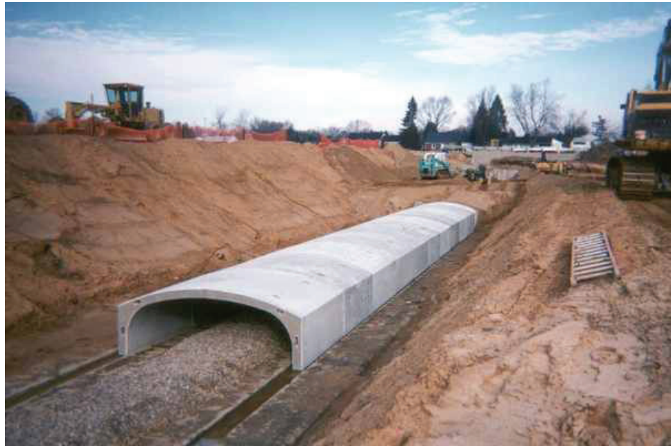
Figure 7.5.4 Precast Concrete Arch with Integral Vertical Legs
