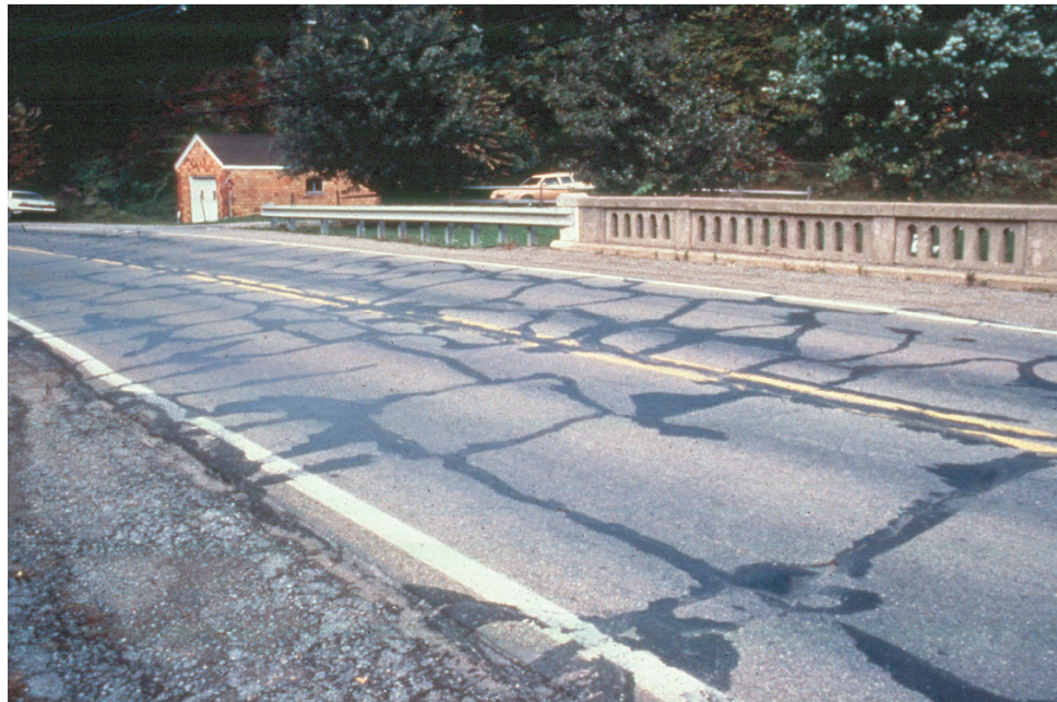
Figure 7.2.17 Asphalt Covered Tee Beam Deck
