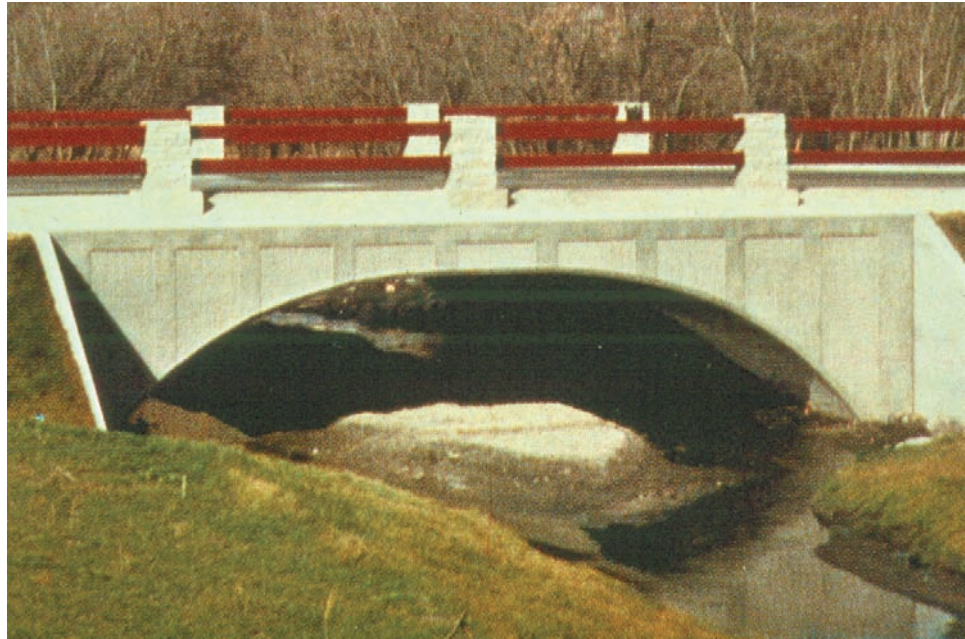
Figure 7.5.7 Concrete Arch Culvert
