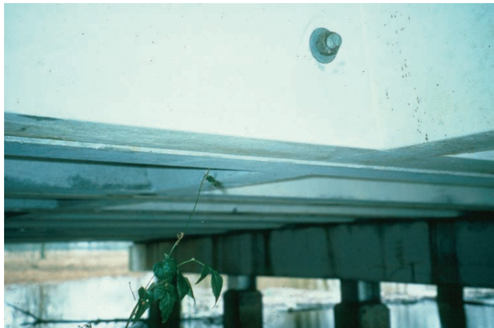
Figure 7.4.8 Stem Tie-bolts
