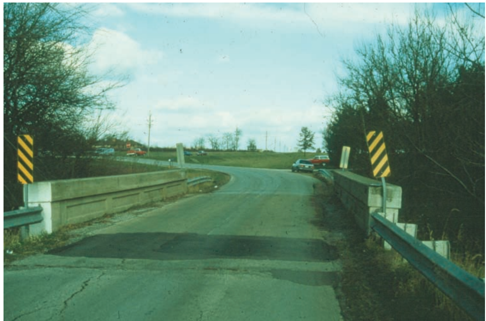
Figure 7.3.2 Concrete Through Girder Bridge
