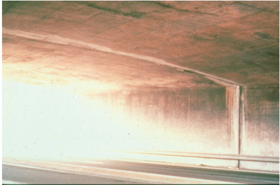
Figure 7.6.15 Longitudinal Joint Between Slab Beam Frames
