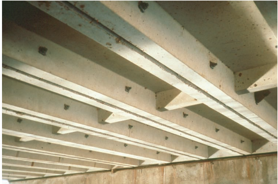
Figure 7.4.1 Underside View of Precast Channel Beam Bridge
