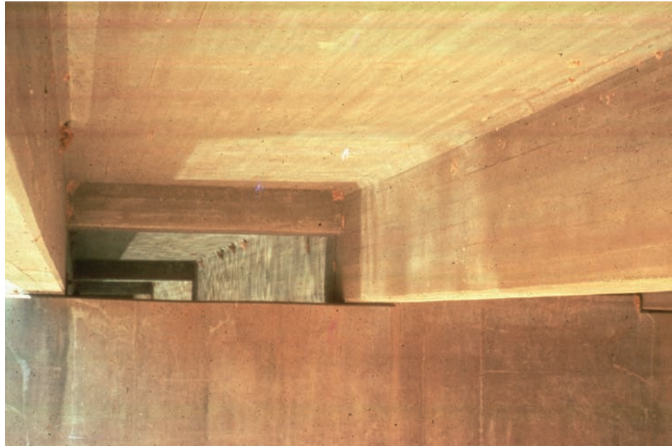
Figure 7.2.6 Tee Beam Primary and Secondary Members
