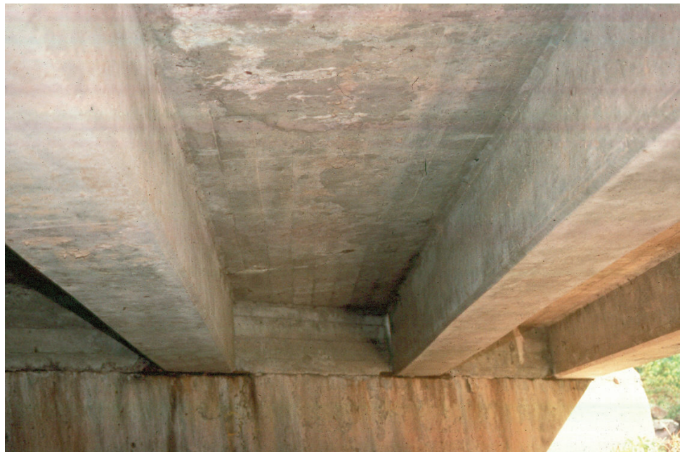
Figure 7.2.3 Typical Tee Beam Layout
