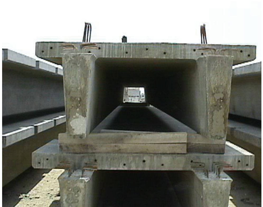
Figure 7.8.1 Typical Prestressed Double Tee Beam
