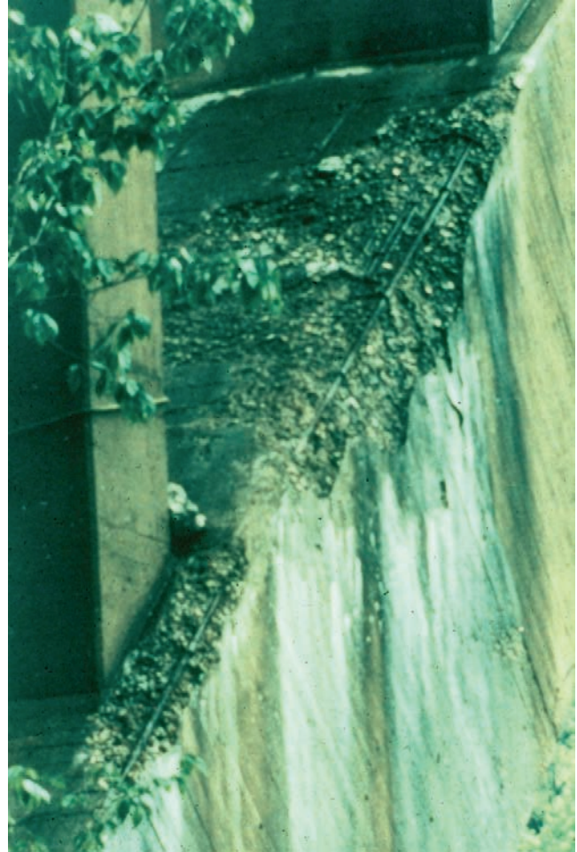
Figure 7.5.18 Scaling and Contamination on an Arch Rib Due to a Failed Drainage System
