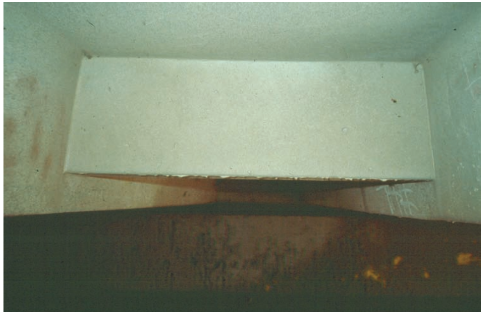
Figure 7.4.10 Close-up of Diaphragm
