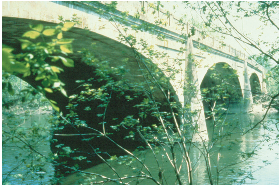
Figure 7.5.2 Multi-span Closed Spandrel Arch Bridge
