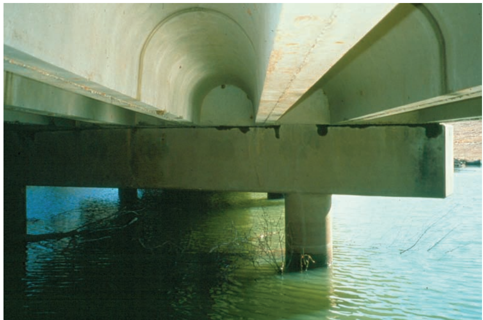
Figure 7.4.2 Underside View of a Cast-in-Place Channel Beam Bridge
