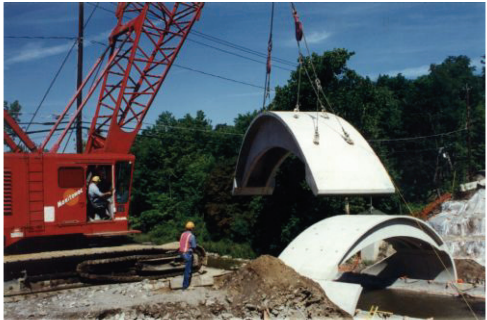
Figure 7.5.5 Precast Segmental Concrete Arch
