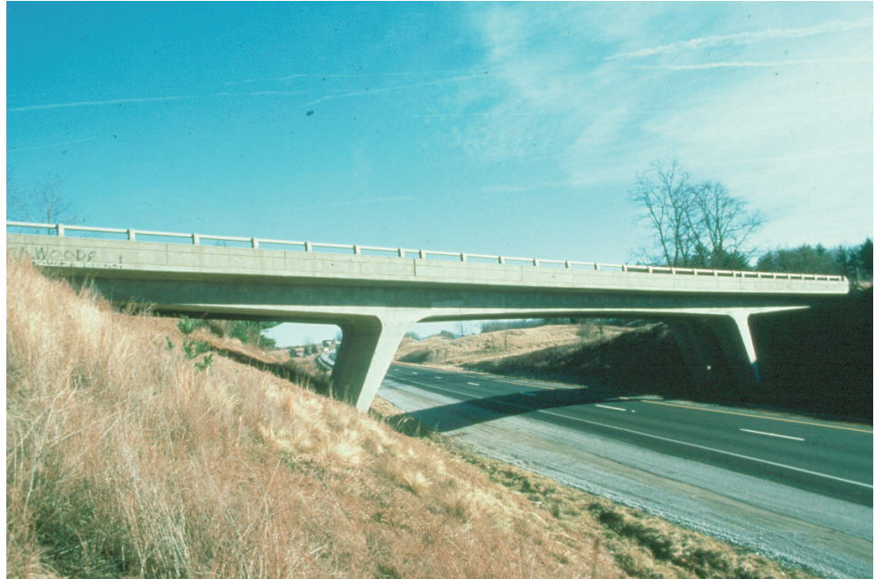
Figure 7.6.4 Typical Concrete K-frame Bridge
