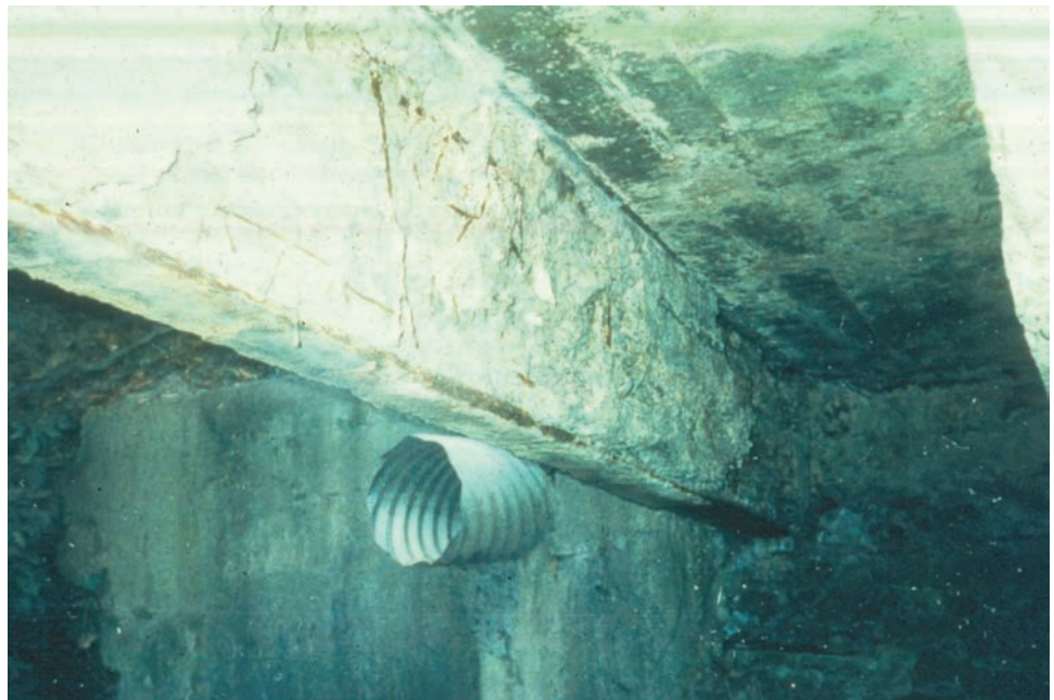
Figure 7.2.5 Concrete Encased Steel I-beam
