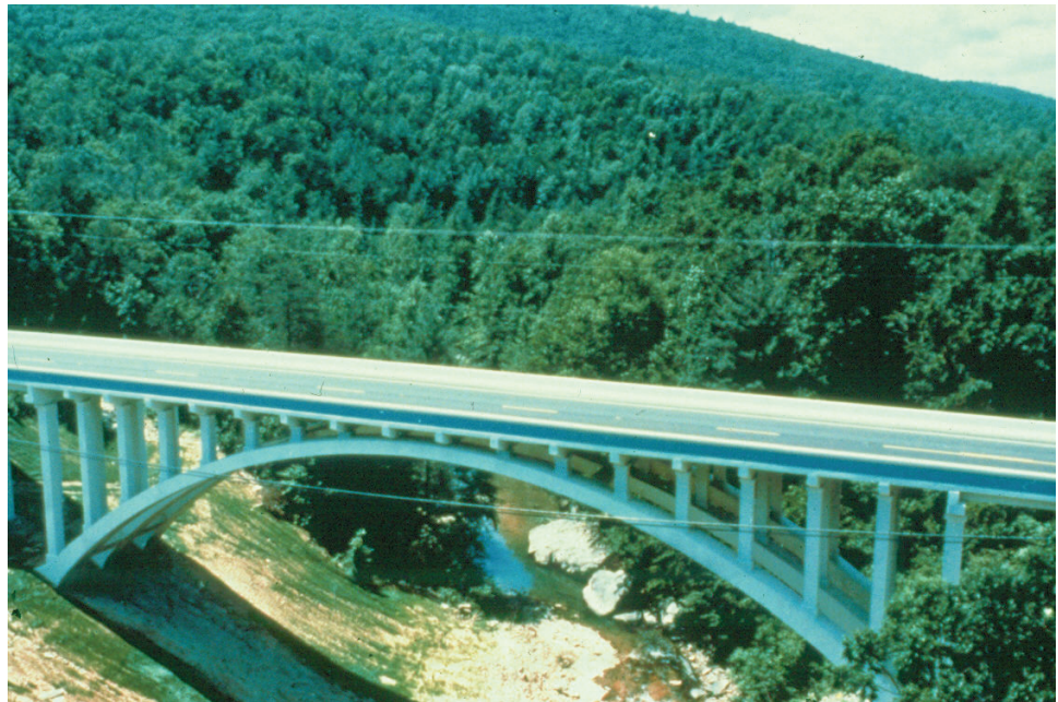
Figure 7.5.1 Open Spandrel Arch Bridge
