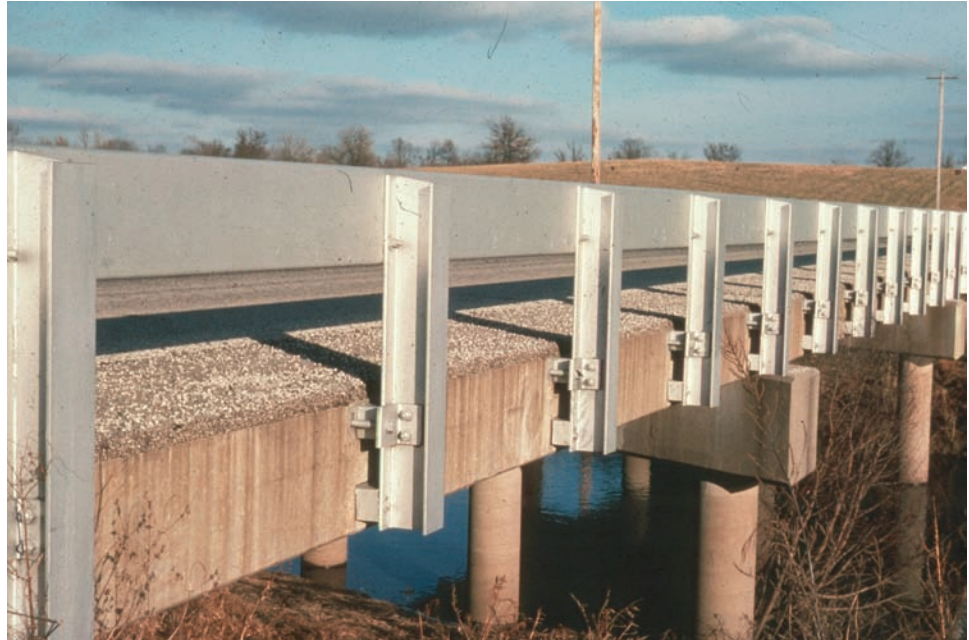
Figure 7.7.1 Typical Prestressed Slab Beam Bridge
