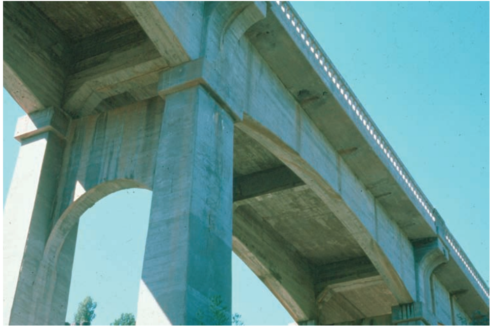
Figure 7.3.3 Concrete Deck Girder, Underside View
