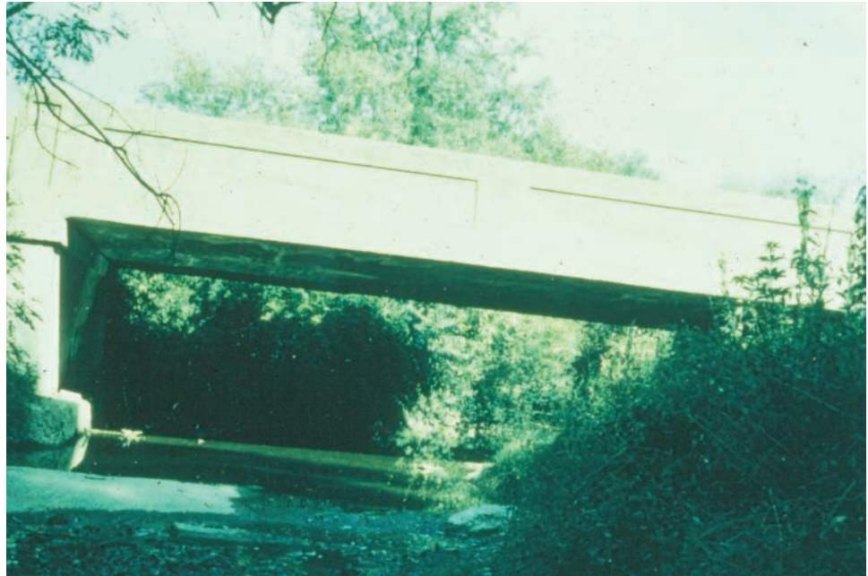
Figure 7.3.4 Concrete Through Girder Elevation View
