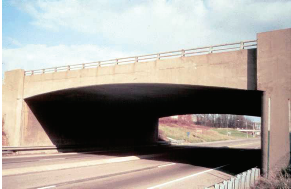
Figure 7.6.2 Typical Single-span Rectangular Concrete Rigid Frame Bridge
