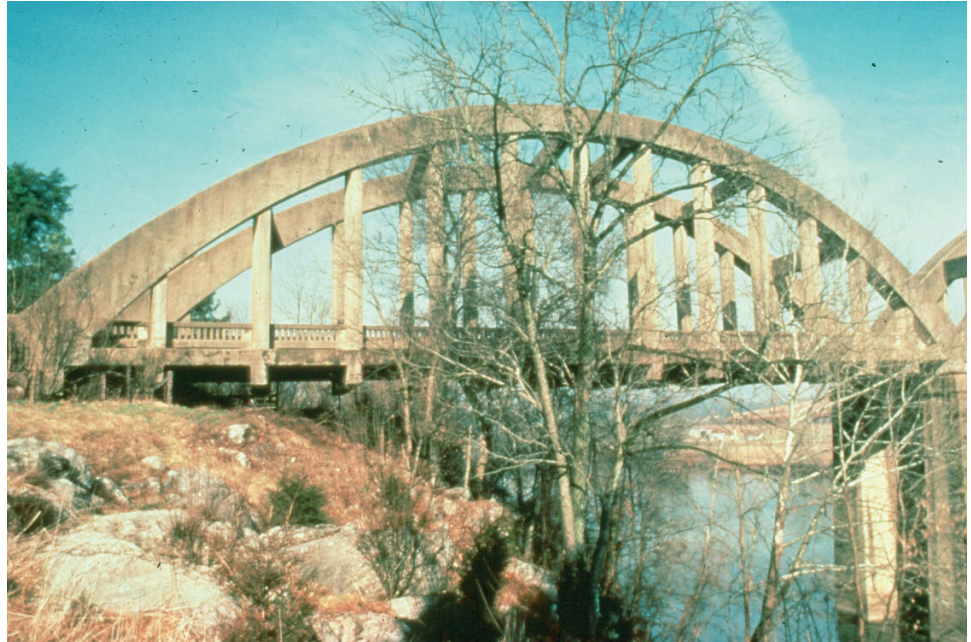
Figure 7.5.3 Concrete Through Arch Bridge
