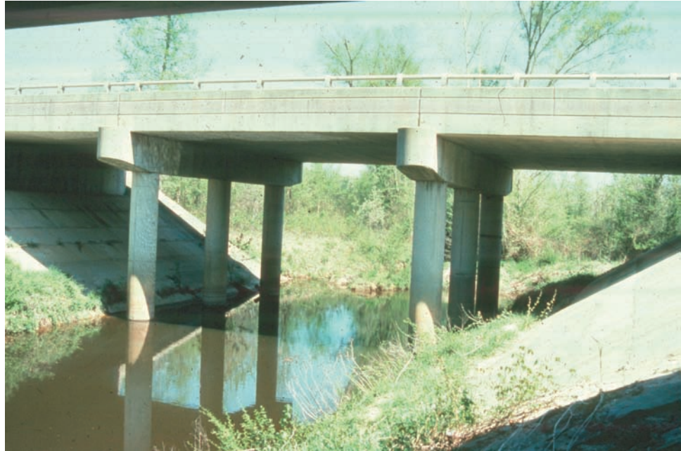
Figure 7.1.2 Typical Multi-span Cast-in-Place Slab Bridge
